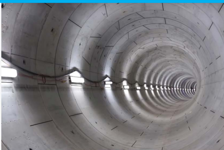
Stamford Diversion Canal and Stamford Detention Tank
